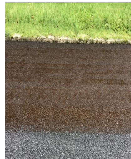
Pictured Above: Fog Seal less than 5 minutes after application
