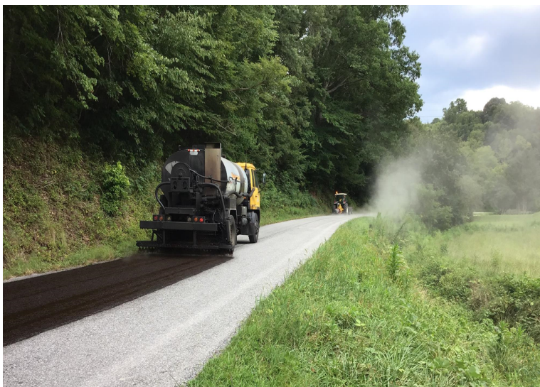
Pictured Above: Cleaning the Road and Fog Sealing
