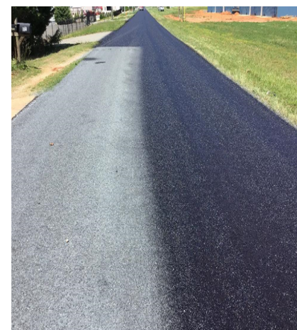
Pictured Above: Fog Seal after emulsion has broken.
